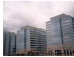
North View Tech Park
