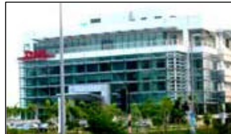
DHL Global Data Center
